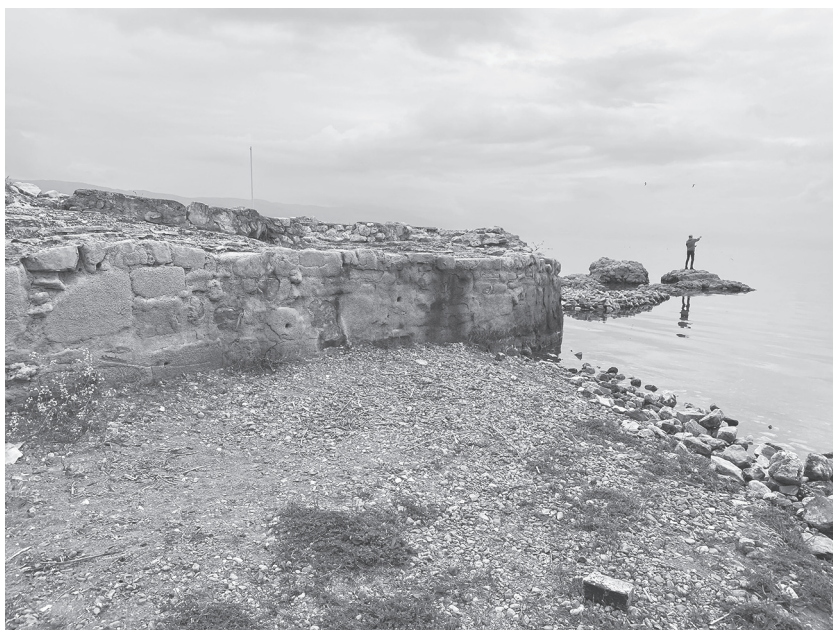
Figure 1.2. Masonry jutting out into Lake Iznik, north of the submerged basilica
